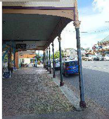
217 DOWLING ST COMMERCIAL AWNING WITH STEEL COLUMNS THOUGHTFUL HERITAGE COLUMNS, PANELS AND DECORATIONS. NO DOWN PIPES VISIBLE.
