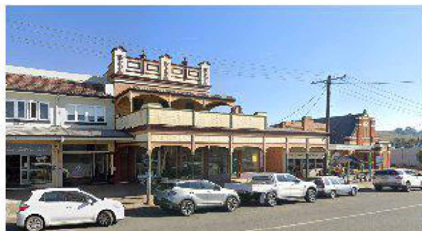
217 DOWLING ST COMMERCIAL AWNING WITH STEEL COLUMNS THOUGHTFUL HERITAGE COLUMNS, PANELS AND DECORATIONS. NO DOWN PIPES VISIBLE.
