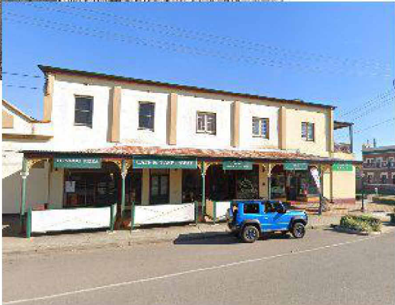
257 DOWLING ST COMMERCIAL AWNING WITH STEEL THOUGHTFUL HERITAGE COLUMNS AND DECORATIONS. STORM WATER DISCREET DISCHARGING AT BUILDING LINE DUE TO ROOF PITCH
