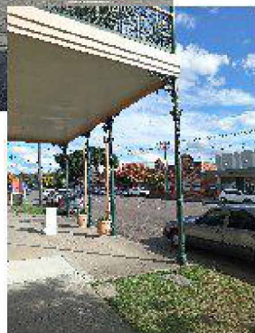
140 DOWLING ST COMMERCIAL AWNING WITH STEEL COLUMNS THOUGHTFUL HERITAGE COLUMNS AND DECORATIONS. STORM WATER DISCREET DUE TO BEING 2 STORIES
