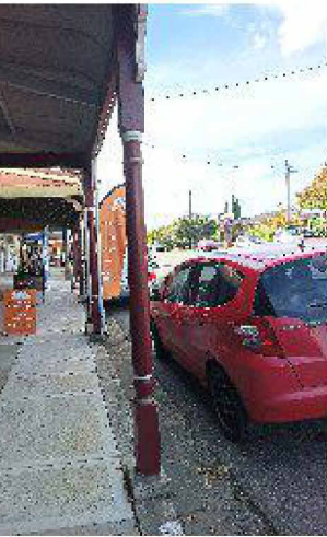
137 DOWLING ST COMMERCIAL AWNING WITH TIMBER COLUMNS THOUGHTFUL HERITAGE COLUMNS AND DECORATIONS. STORM WATER DISCREET DISCHARGING TO STREET KERB
