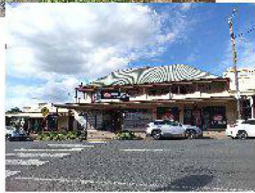
227 DOWLING ST COMMERCIAL AWNING WITH STEEL COLUMNS THOUGHTFUL HERITAGE COLUMNS AND DECORATIONS. STORM WATER DISCHARGES TO STREET KERB
